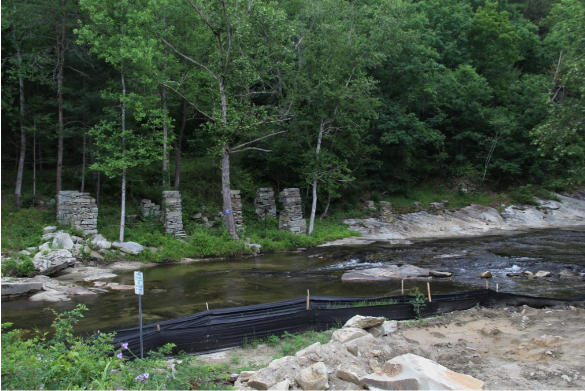
Brewer's Mill site, view to northwest
