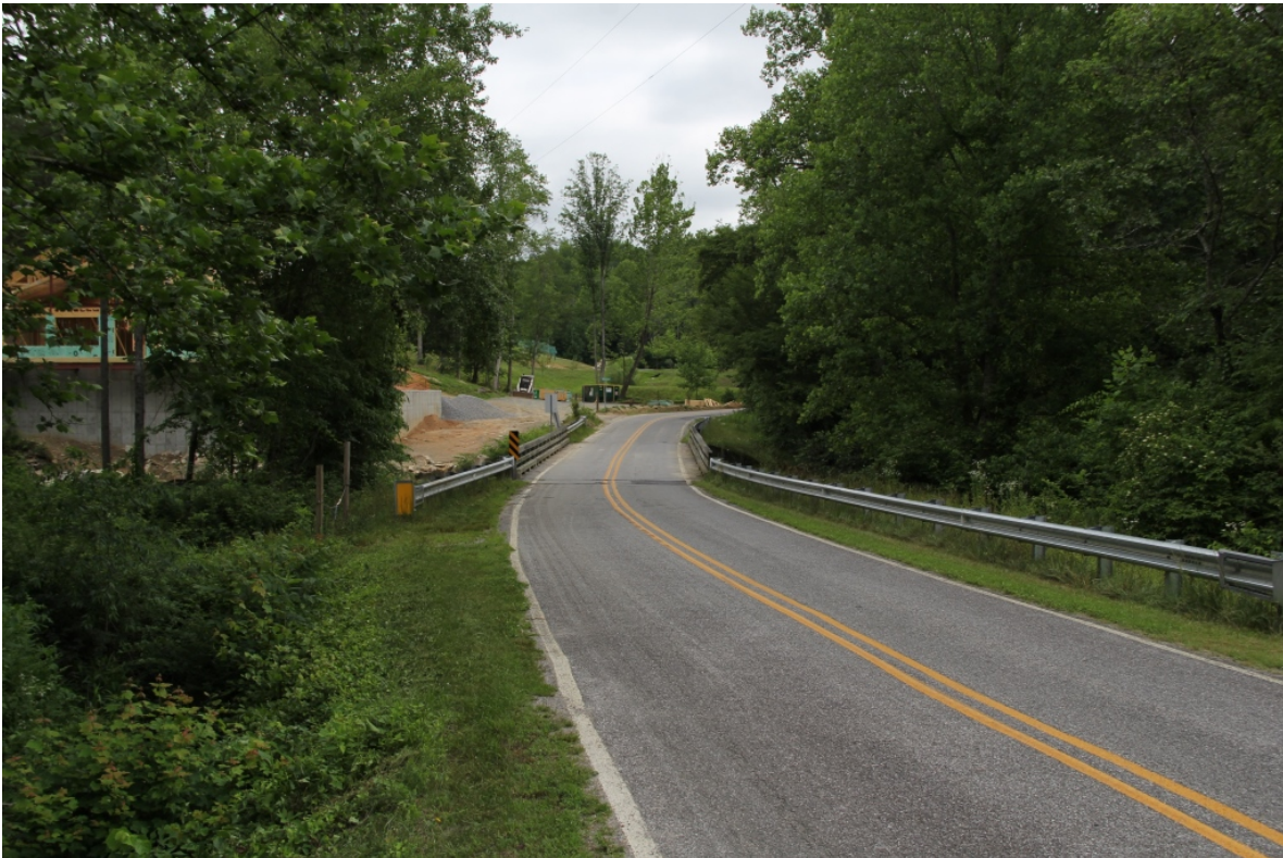
Bridge No. 436, view to east along Brewer Mill Road (SR 1943)
