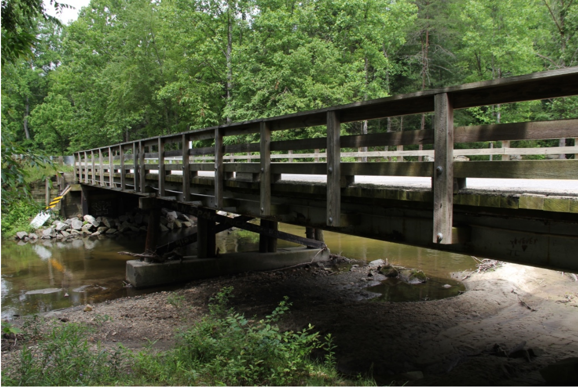
Bridge No. 436, oblique view to northwest
