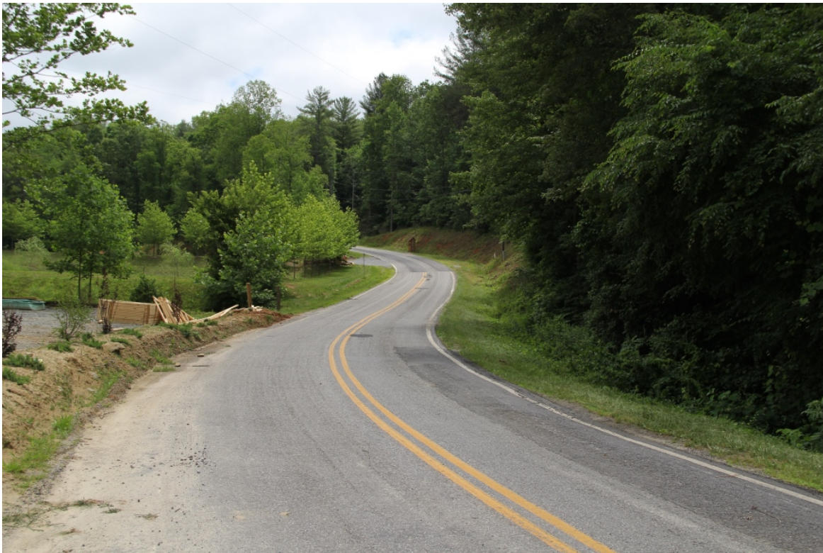
View to east along Brewer Mill Road (SR 1943) from east end of Bridge No. 436
