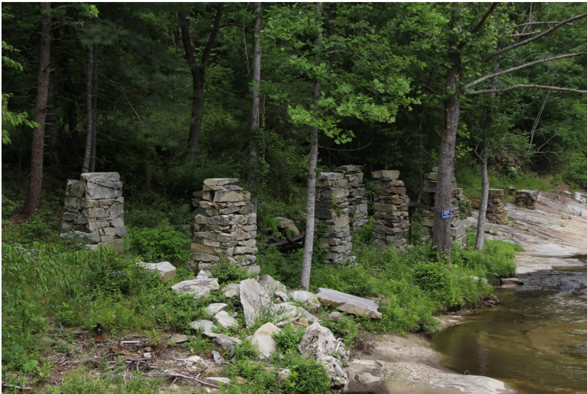
Brewer's Mill site, foundations, view to north
