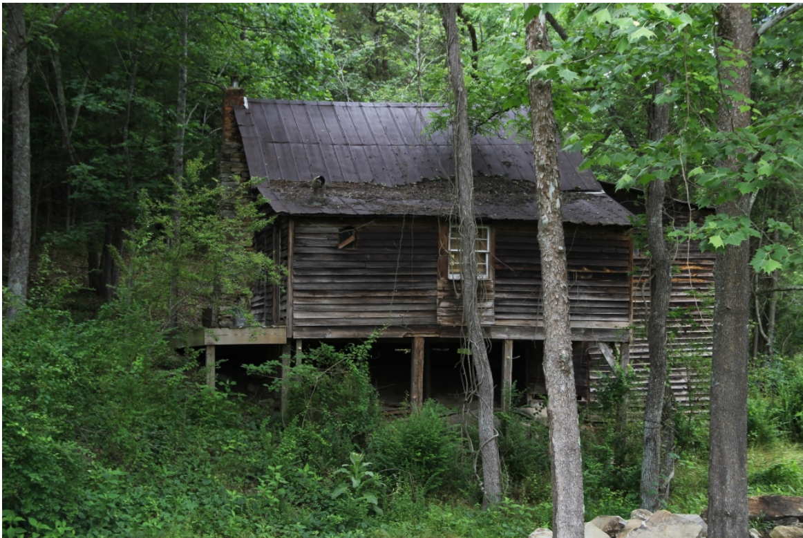
Miller's House, 447 Brewer Mill Road, view to north
