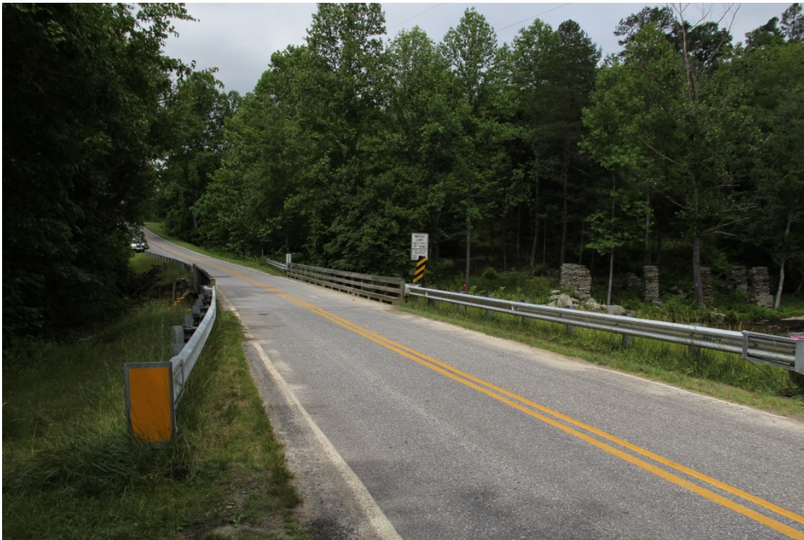
Bridge No. 436, view to west along Brewer Mill Road (SR 1943)
